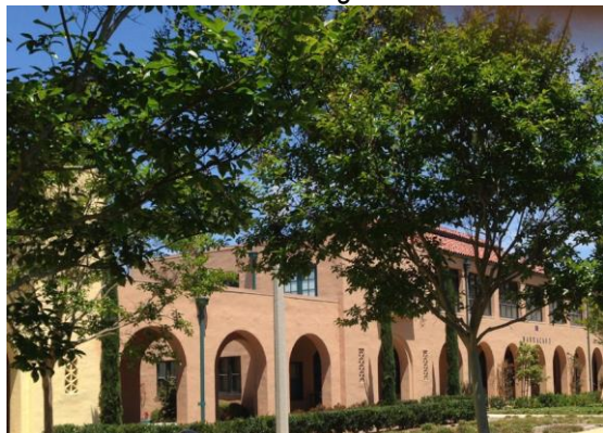
Repurposed barracks at the Naval Training Center, now part of the complex called Liberty Station.
