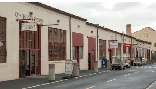
Photo of Fort Mason courtesy of National Park Service.
